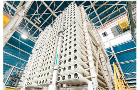
Figure 2: Reverse Osmosis technology selected for the TKO Desalination Plant
