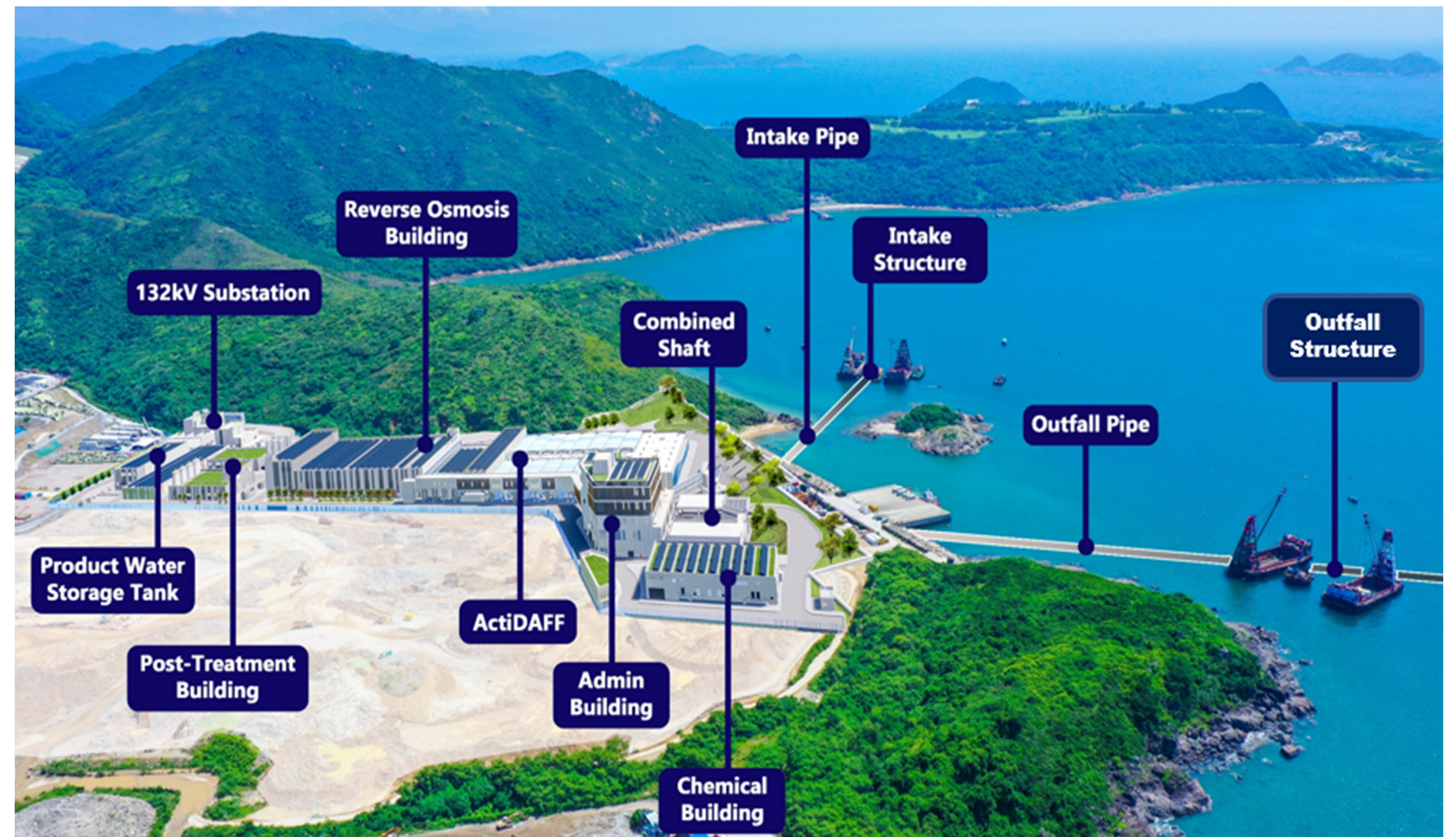
Figure 1: First Stage TKO Desalination Plant
